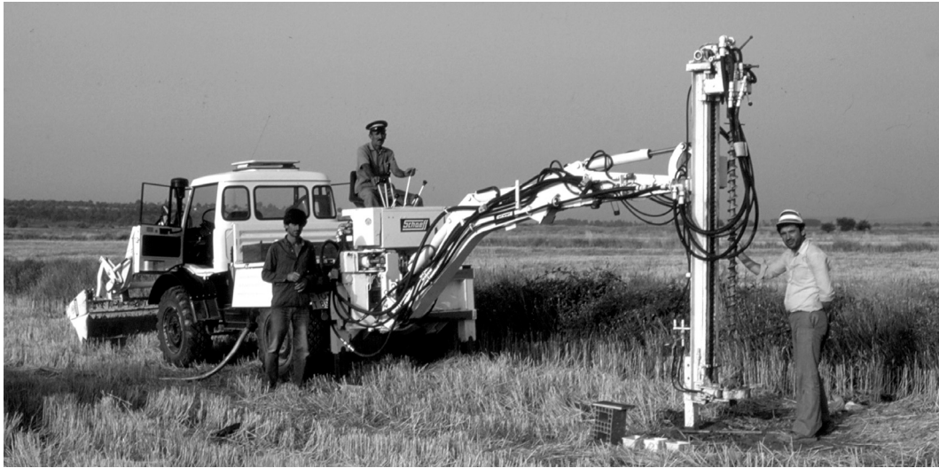
Fig. 9 A screw-drilling operation with Unimog to the north of Troia.
